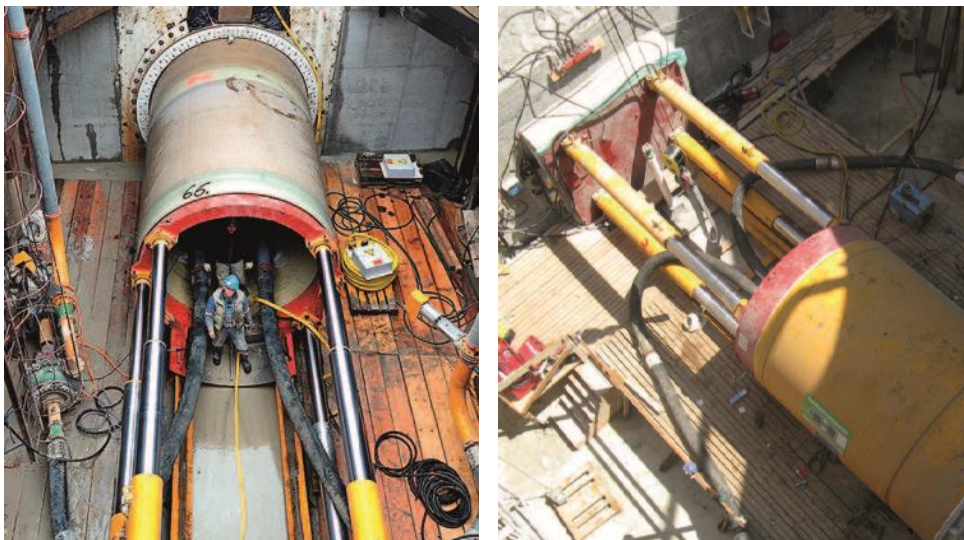
Figur 8-6. Startschakt, s.k. jacking-shaft.
