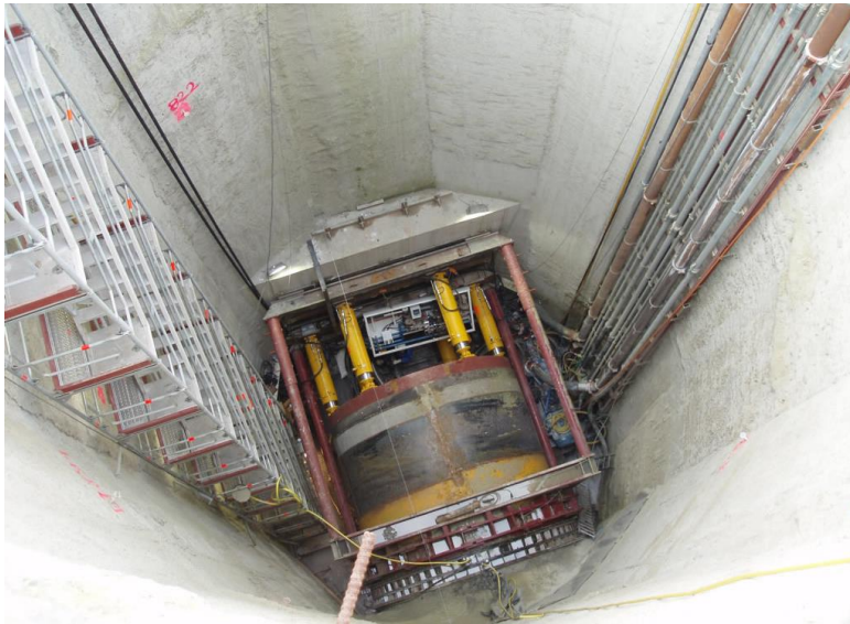
Figur 8-6. Startschakt, s.k. jacking-shaft.
